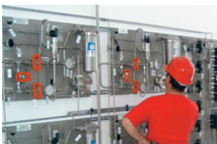
Fast loop panel installation
